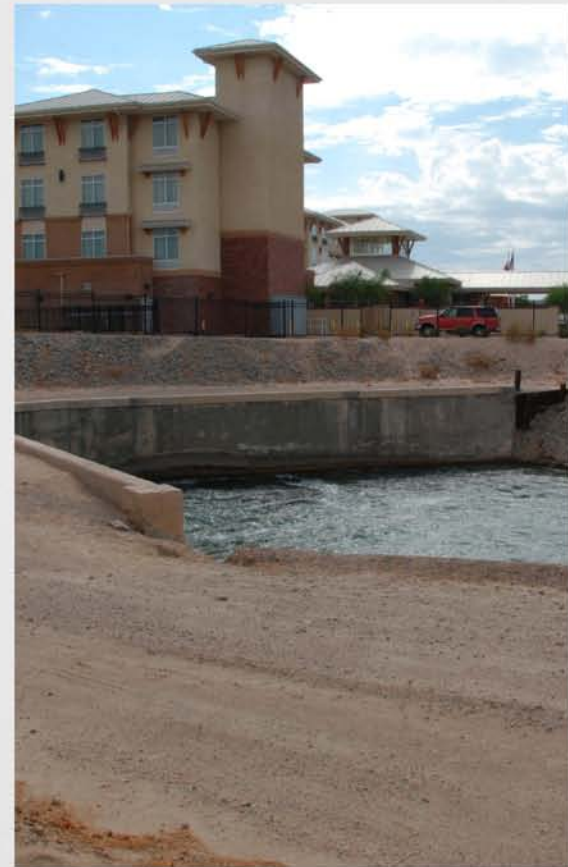
Outlet of the inverted siphon
