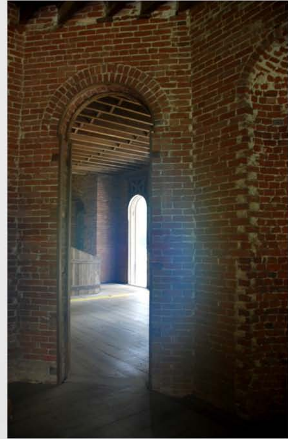
Special 5 sided brick were made for the octagonal design
